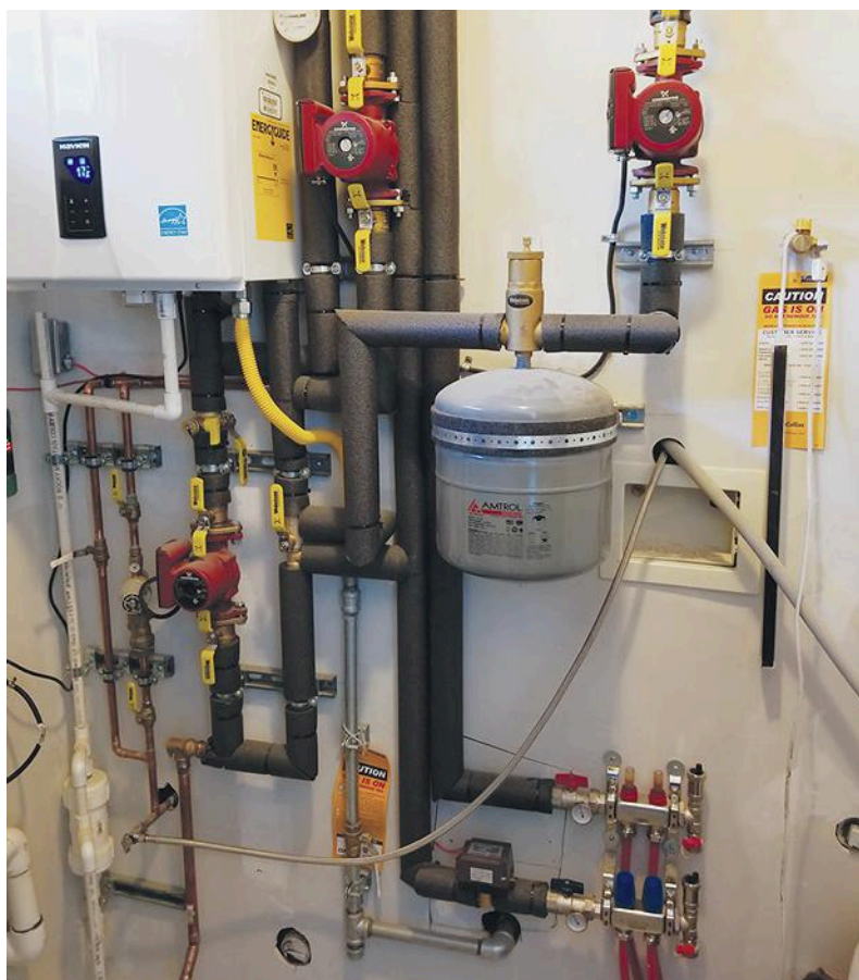
Grundfos UP series pumps (in red) keep water circulating efficiently.
