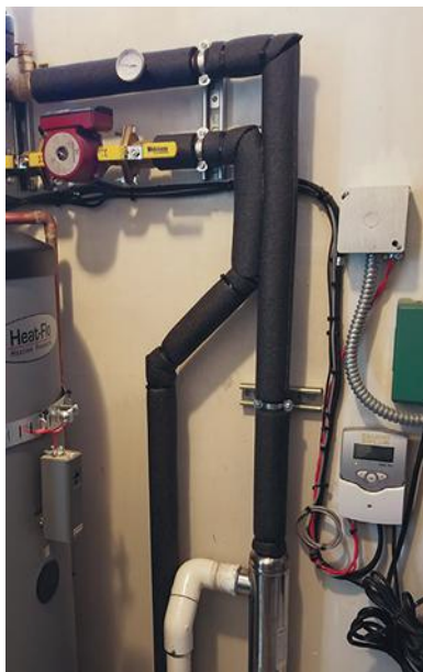
At right you can see part of the control set-up, which includes a Caleffi iSolar Plus unit.
