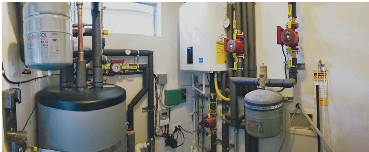
The guts of the system are a Navian NHB 150 mod/con boiler (white box, center) and a Heat Flo HF 60-D 60 gal. dual-coil storage tank (large gray cylinder at left).
