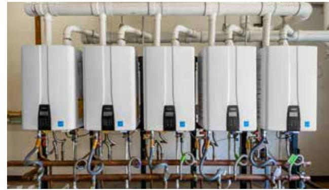
Five NPE-2 Tankless Water Heaters were installed with the Ready-Link Manifold System.
