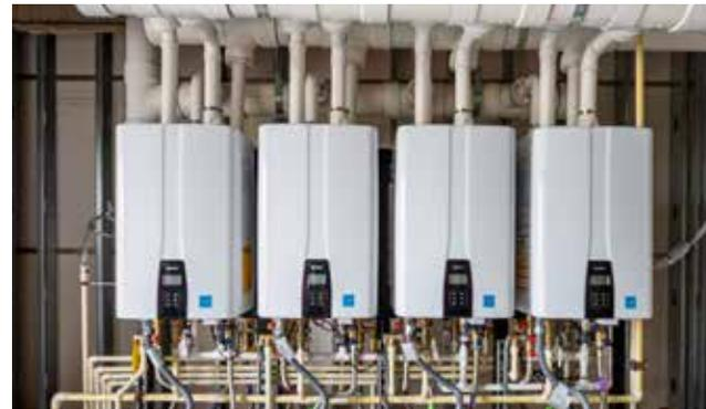
Eight Navien NPE-A2 Tankless Water Heaters were installed with the Ready-Link Manifold System.
