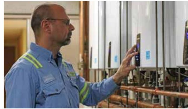
Kevin Berry from KMB had to adjust the temperature setting for each set of tankless water heaters to fit the two supply temperatures needed.
