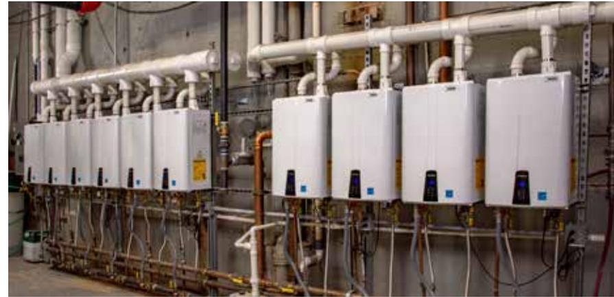
10 NPE tankless water heaters replaced a failing 1.9 million BTU/H boiler to indirect tank system.
