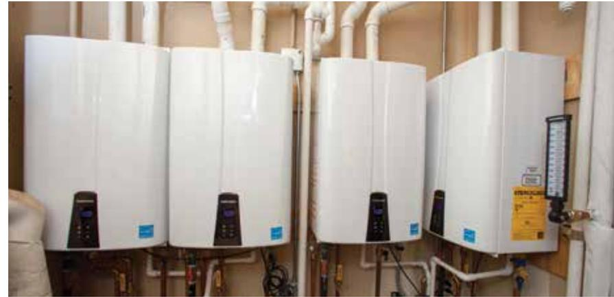
Four Navien NPE-240 units use cascading technology to assure a steady and dependable flow of hot water.
