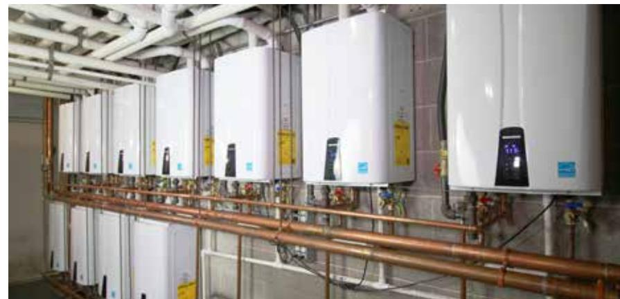
11 cascading Navien NPE-240A units provide endless hot water to the 137-bed facility, complete with commercial kitchen and laundry.
