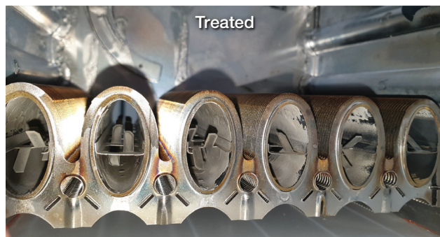
Tankless water heater heat exchanger
